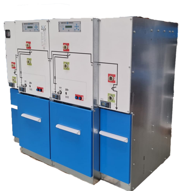
fig.6. DR-6D RMU with RP800 Protection Relay
