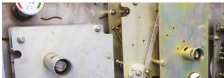
A RV 53 Load Break Switch & Earthing Switch B Mechanical Drive
